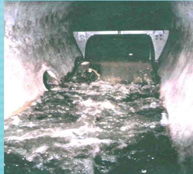
Sewer flushing
